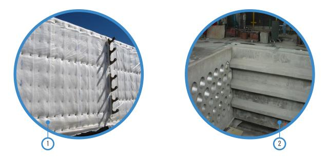
Refractory is used throughout the inside of the heater to shield the heater casing from excess temperatures. It is typically designed to reduce the outside temperature of the metal casing to 180° F (per API 560 specification). There are many different types of refractory, but the most common types are castable and ceramic fiber.
